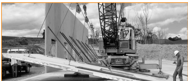
Props attached prior to lift
