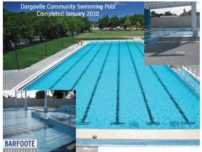
The finished result! A 50m length swimming pool that the whole community can be proud of.
